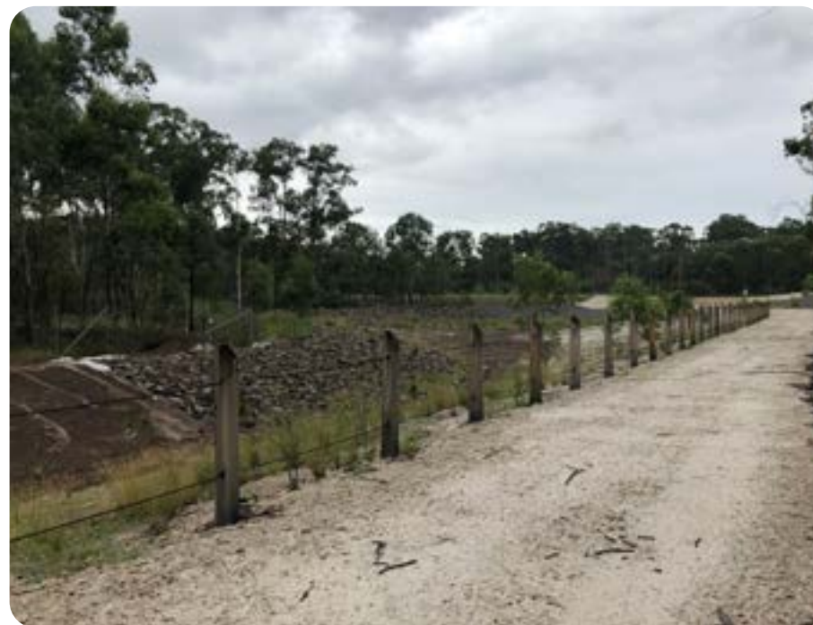
View 5: Existing Open Drainage Channel
