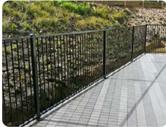
Tubular Fencing (1.2m Safety Fence)
