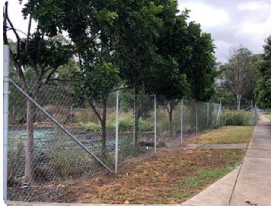
Existing fences along Jordan Spring Boulevard
